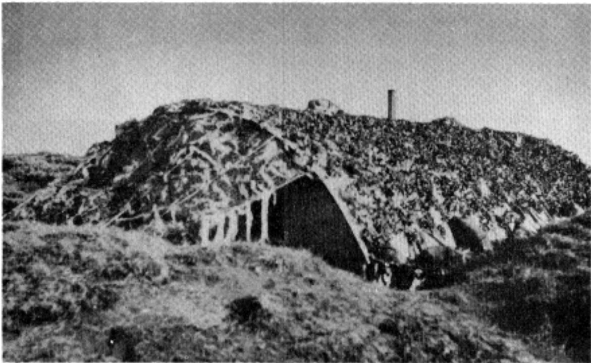
Figure 59. Here is a quonset hut blended into the terrain by a combination of digging in, texturing, and covering with a net.
